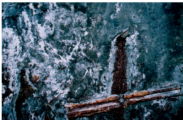
Fig. 7. Salt accumulations (principally thenardite with subordinate gypsum) on the walls of the Cruachan underground power station, Scotland. (Width of field of view c. 1 m). These sulphate salts have formed by evaporation to dryness of groundwater entering the facility, in which the air is heated by operation of hydro-power turbines. (Note the small seepage of groundwater (dark in colour) from a former rock-blot hole, and the badly corroded face plate in the lower right of the field of view; these illustrate the challenge of salt-assisted corrosion in underground voids maintained open for several decades.)
