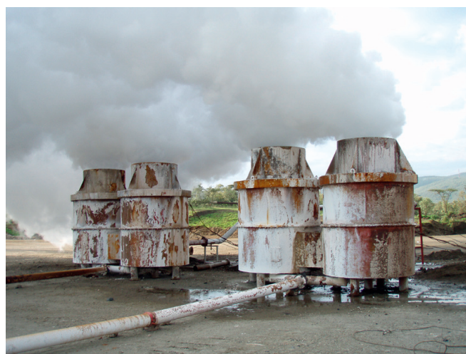
Fig. 4. Typical amorphous silica precipitates (white staining) at active high-enthalpy geothermal wells in the Rift Valley, Kenya, on 23 May 2012. (a) Silica scale on wellhead valve work and in the borehole cellar at Menengai No. 1 Production Well (capacity 8 MW e ) of the Geothermal Development Company of Kenya (location: UTM zone 37M; Northings 9976800m; Eastings 171850m). (b) Silica scale on four steam–water separators, silencers and water removal pipelines serving the Olkaria No. 11 Production Well (capacity 9.6 MW e ) of KenGen (location: UTM zone 37M; Northings 9900850m; Eastings 200240m).
